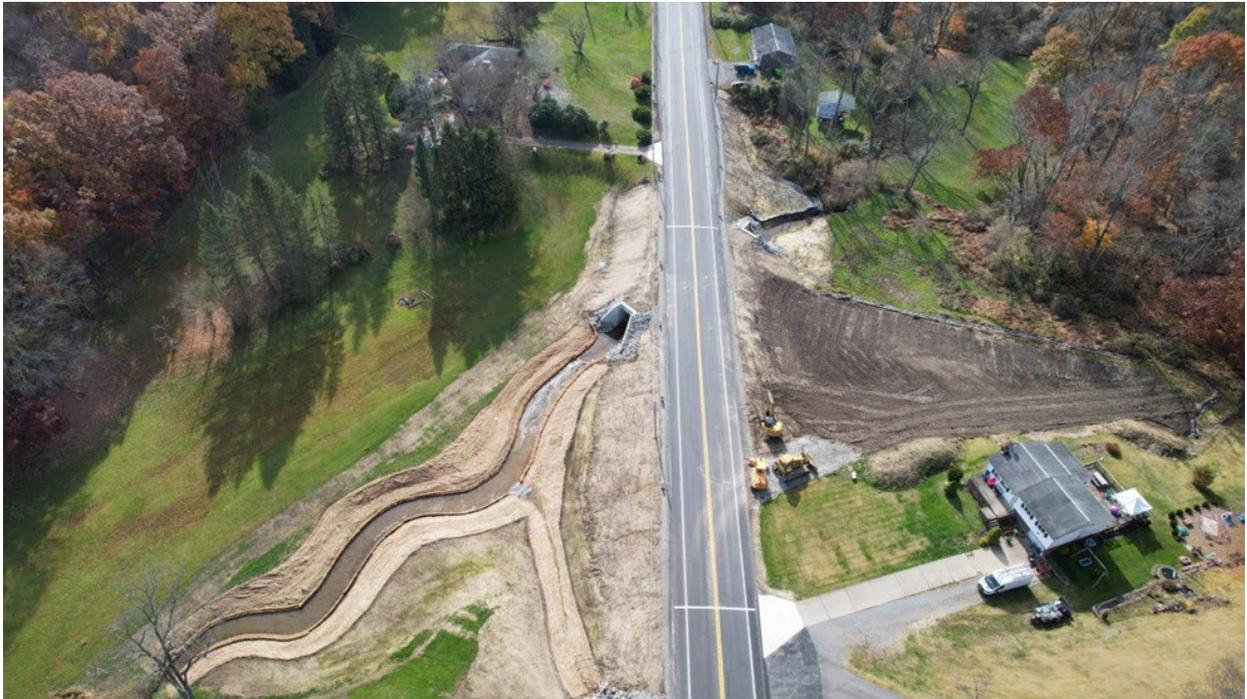
Photo 2: Newly constructed precast concrete box culvert carrying SR 356 over Tributary 2 to Kiskiminetas River
